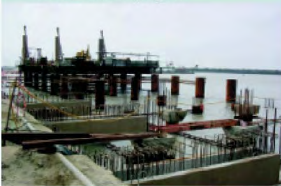
New berth under progress
