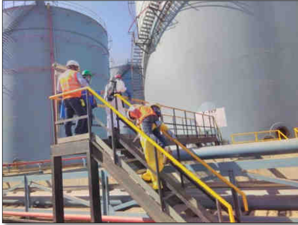
Incident Spot : Inside Liquid Terminal (Enclosure-09, Tank no. 117)
