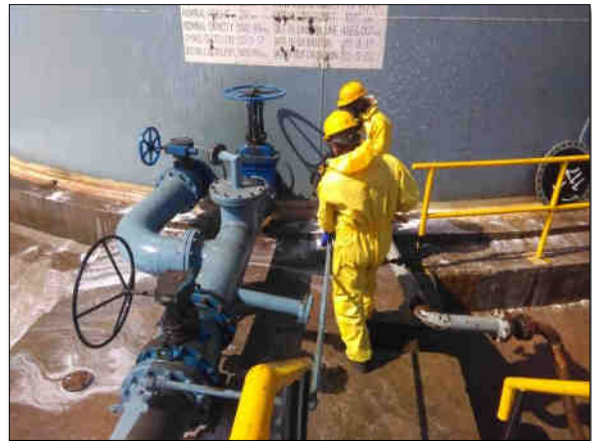
Maintenance staff reached at site
