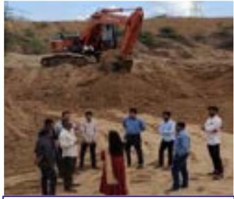
Restrengthening & Desilting of Check dam – 720+ Benefited
