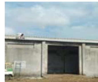
3 Villages - Renovation of Godown and Gauthala Shed
