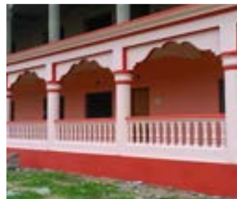
Renovation of High School at Zaarapa – 2200+ Benefited
