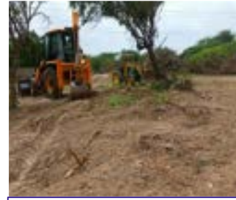
River Cleaning and JCB Support - 2250+ Benefited
