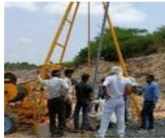
6 Percolation Bore well Recharge – 4000+ Benefited
