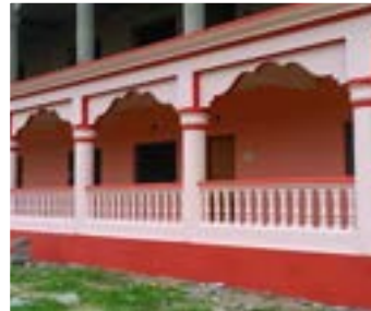
Renovation of High School at Zaarapa – 2200+ Benefited
