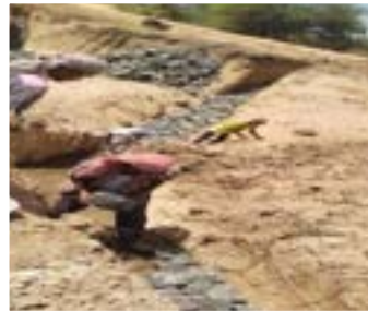
Construction of Pipe Culvert – 400+ Benefited
