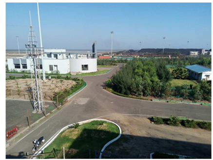
Near SS-01 Building
