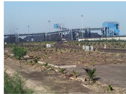
Near SS-02 Building
