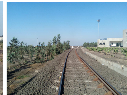
Near Railway Building
